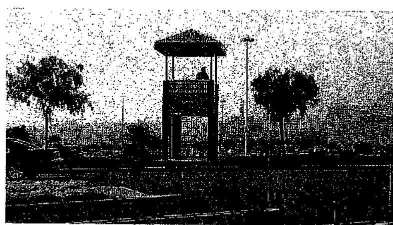
Figure 10.4. Security watchtowers at the TownGate Mall in Moreno Valley. (Photograph: A. Jonas)
