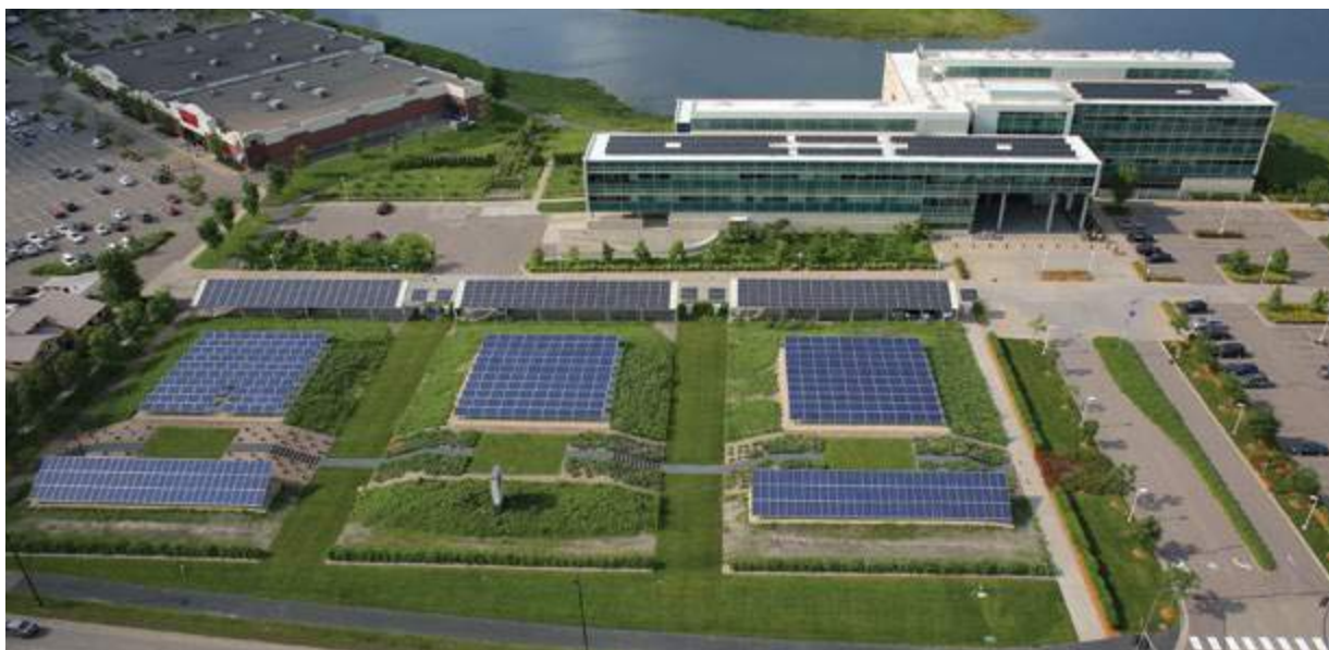
Great River Energy's headquarters site will test a variety of solar technologies and configurations. The new 250-kW installation expands upon 72 kW of solar panels that were installed in 2008. The array includes panels made by Sharp (two rows pictured at bottom), tenKSolar (three square-shaped clusters) and Suniva (three rows closest to the building).
